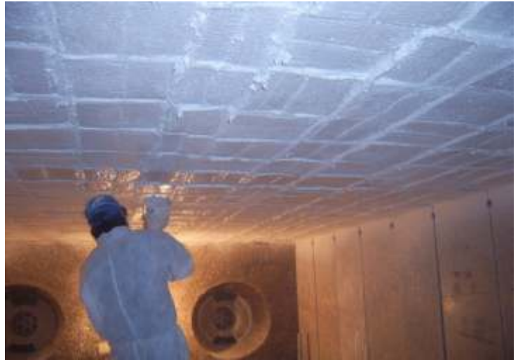
Forge Industry Refractory lined with Ceramic fibre Pyrobloc
